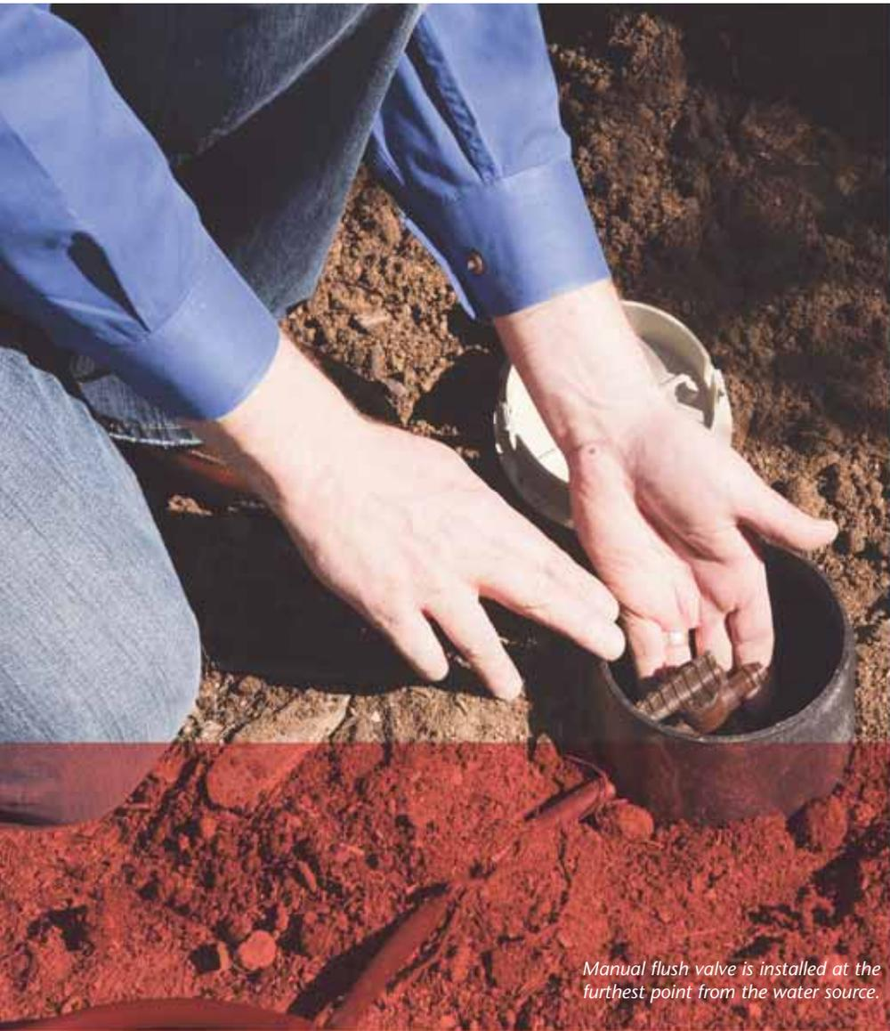
*Manual flush valve is installed at the furthest point from the water source.*
