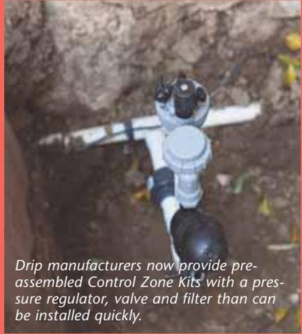
*Drip manufacturers now provide pre-assembled Control Zone Kits with a pressure regulator, valve and filter than can be installed quickly.*
