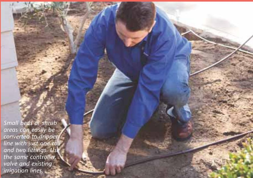
*Small beds or shrub areas can easily be converted to dripper line with just one roll and two fittings. Use the same controller, valve and existing irrigation lines.*
